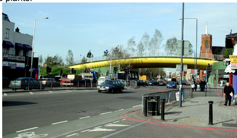
The Green Bridge
